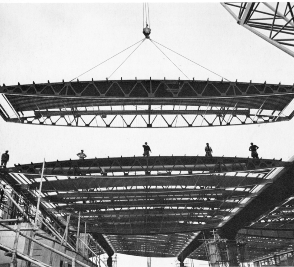
Top: While the structure of the Osaka Prefectural Sports Center is being erected, panels are being assembled on the ground nearby.
